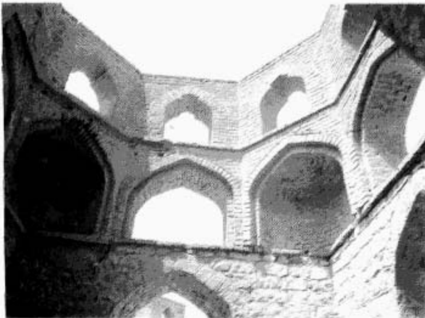
62. The square lower storey and the zone of transition in the mausoleums of the seven domes.
